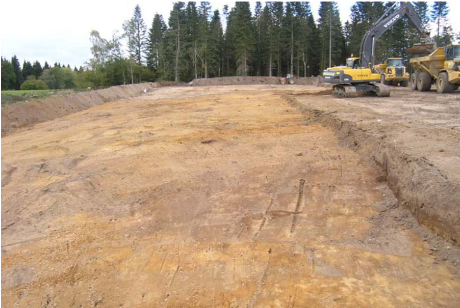
Plate 5: Exposure of natural deposits 102 during removal of former ploughsoil layer 101.
