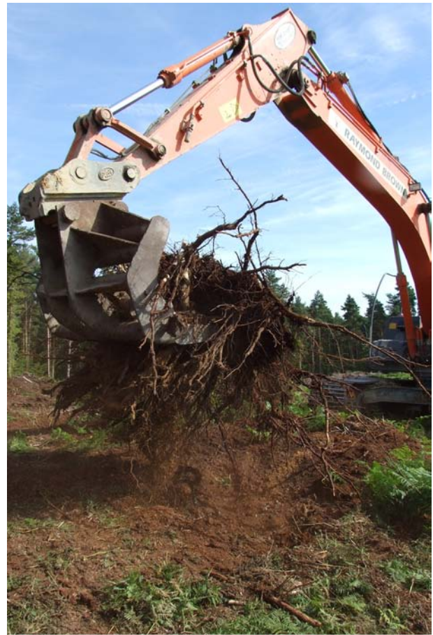
Plate 3: Removal of tree stump – shaking soil from the roots.
