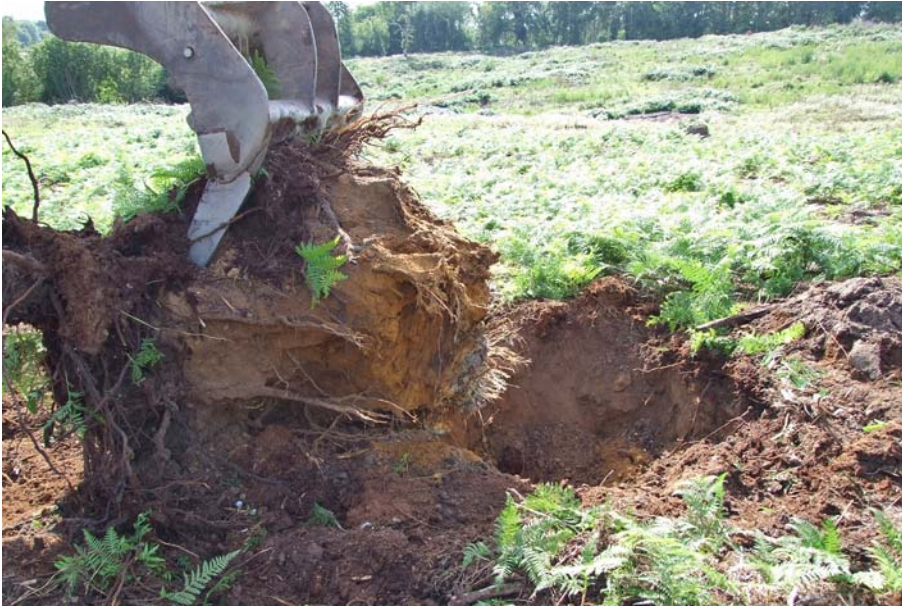
Plate 4: Detail of typical medium-sized tree stump being extracted.
