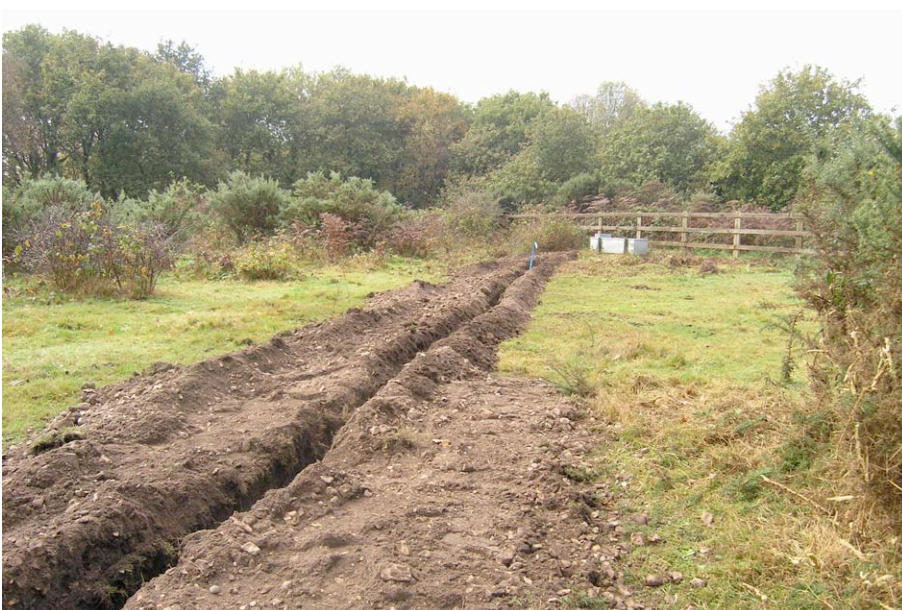
Plate 3: View of southwestern end of the pipe trench.
