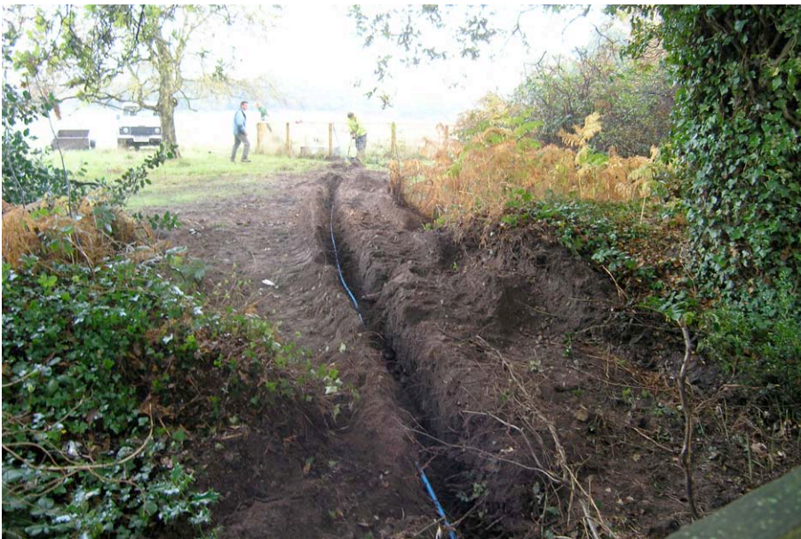
Plate 2: View of northeastern end of the pipe trench.
