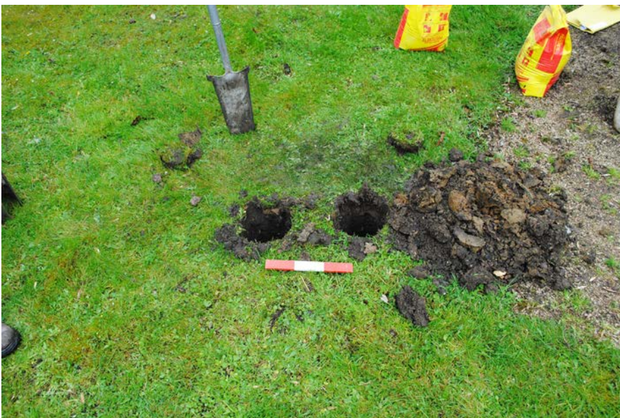
Plate 3: Post holes for new interpretation panel, looking south. 0.3 m scale.
