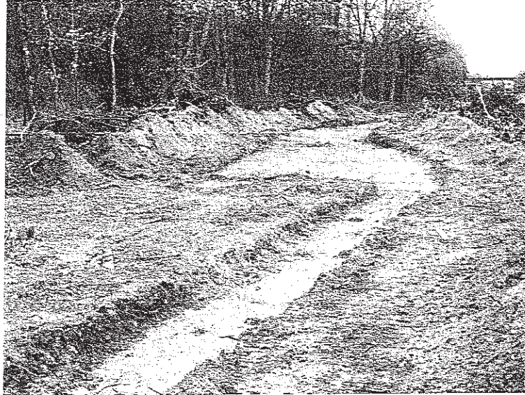
Plate 8. General view of excavations at Site 3 – Millfield Plantation
