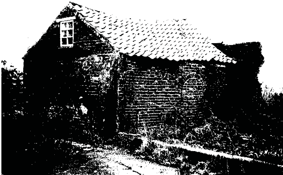
Plate 2. Loosebox to the rear of Georgian House, from the south
