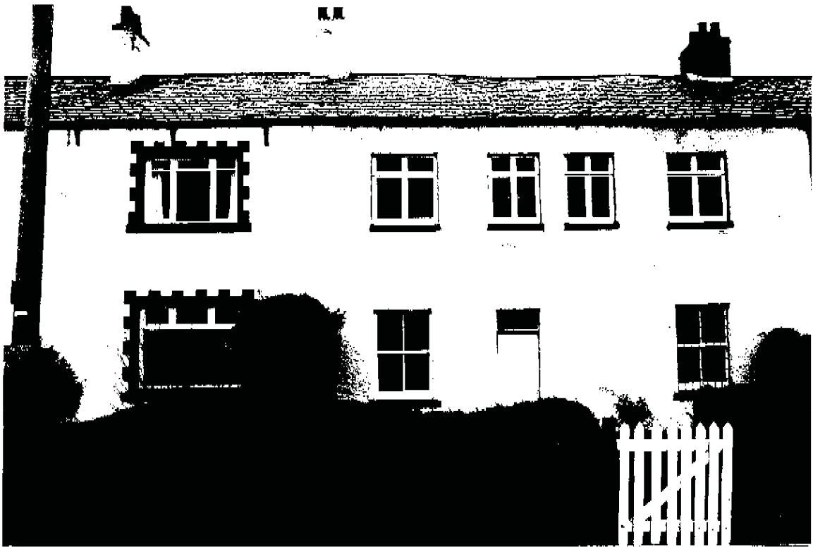
Plate 3. No 1 Hopetown Terrace (bay 4) from the west
