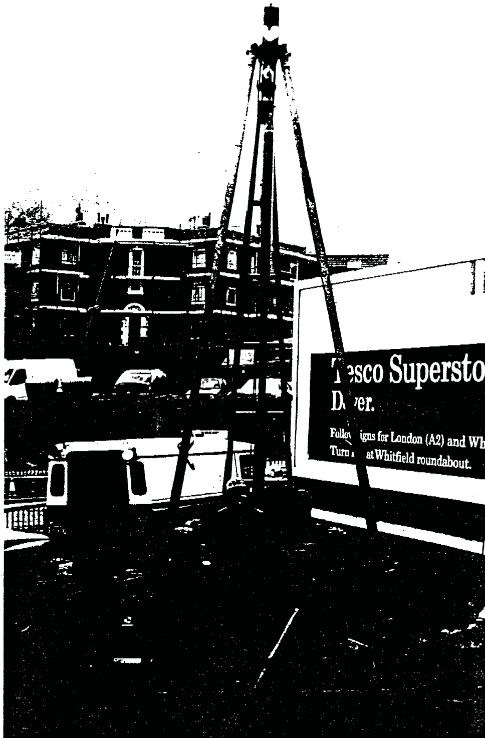
Plate 2. Shell and auger drilling at the Crypt site (DS-C), Dover
