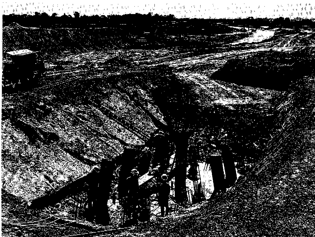
Plate 34 Area 2 during construction of the Bypass
