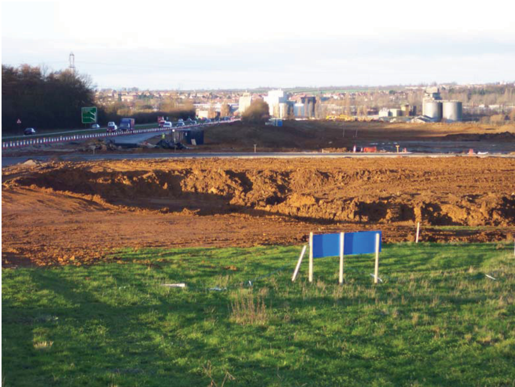
Plate 1: New road, joining the A45. Facing west towards Wellingborough
