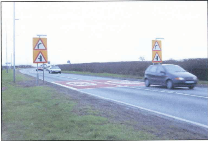
Plate 2 (right): Signage Pit S1, looking northeast.
