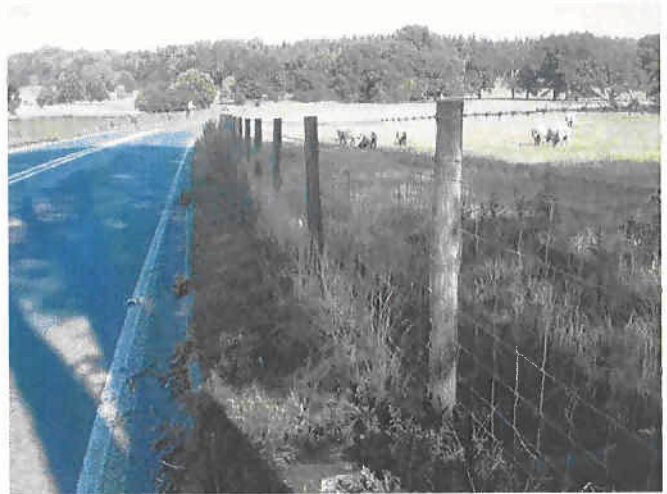
Plate 2: Post-and-wire fence on east side of A49
