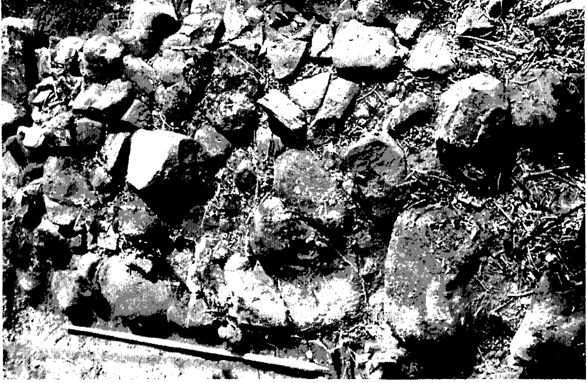
Pl. 2. Site 38, Trench B looking north-east. Wall 2007 is to the left with the later addition, Wall 2009, to the right.
