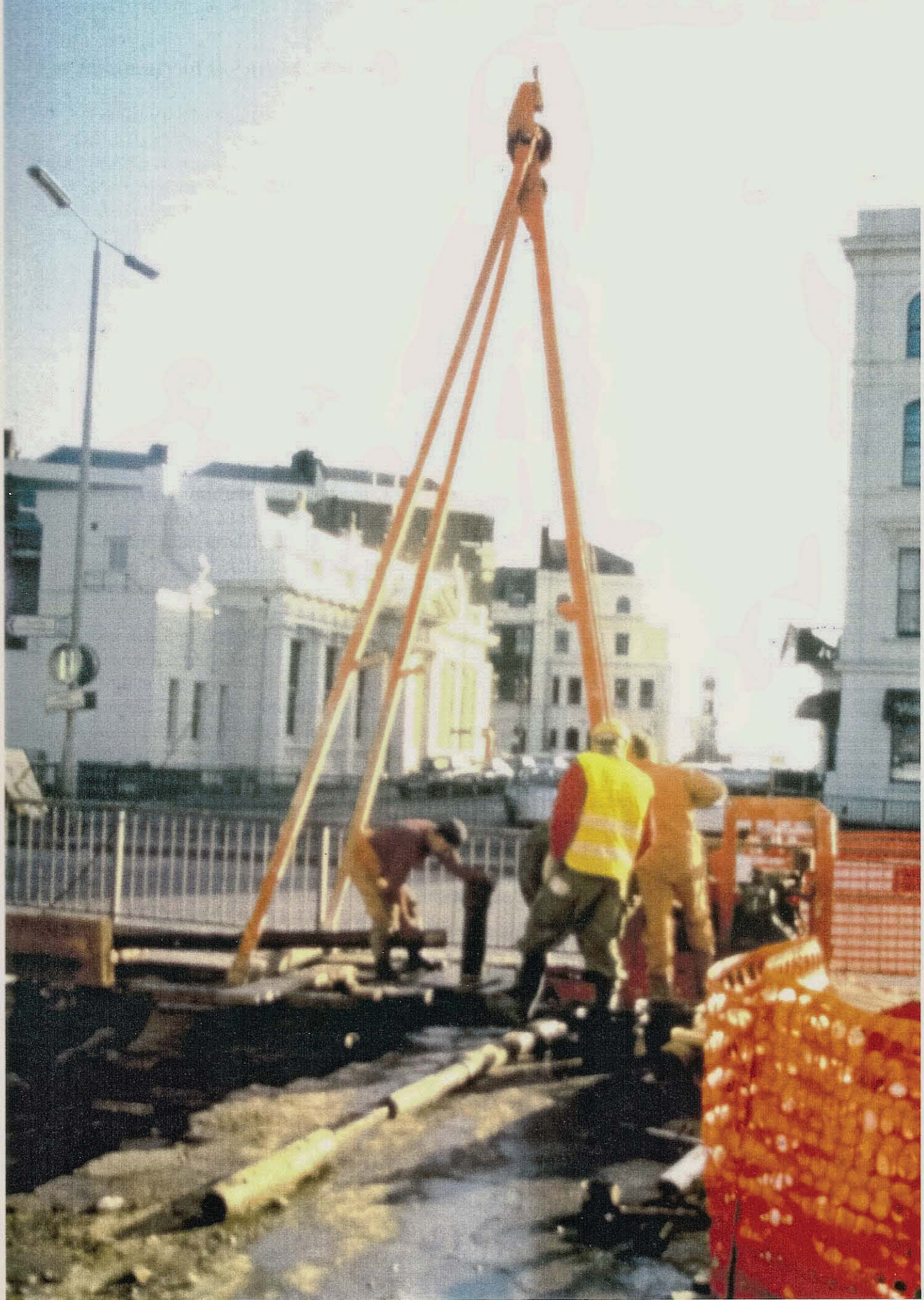
Fig. 4 Taking core samples at the end Bench Street.
