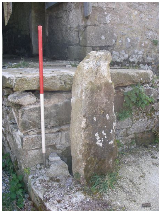
Plate 3 Granite gatepost with wedge marks (north of Building 3).
