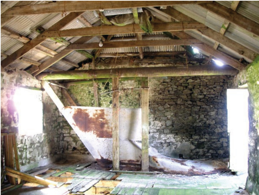
Plate 4 Inserted hopper on the first floor of Building 3.
