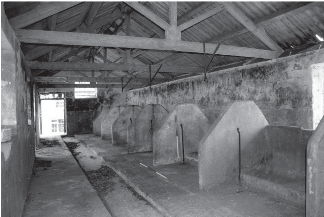
Plate 5 Building 5 cow stalls looking east, showing the gabled slate roof structure including tie beams, king post and principal rafters braced with struts.
