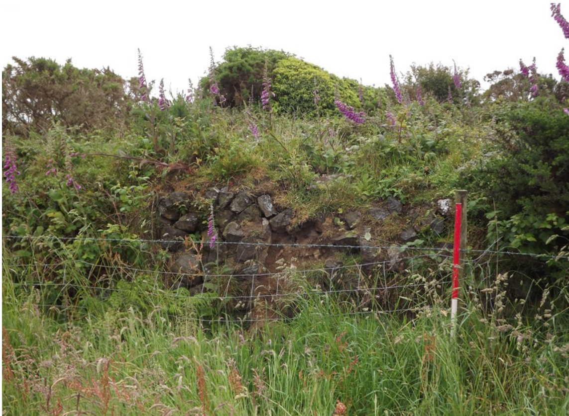
Plate 5 Representative section of Proposed Turbine Field boundary. Looking east.
