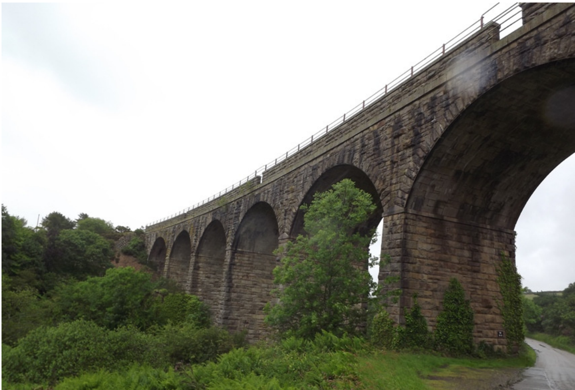
Plate 9 Blackwater Railway Viaduct (Site 92). Looking southeast.
