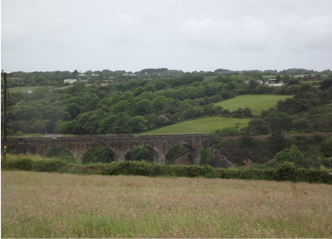
Plate 8 Blackwater Railway Viaduct (Site 92) from Proposed Turbine Field. Looking north.
