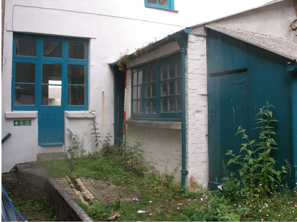
Plate 4 Outbuilding [9] centre and outbuilding [10] right, looking northwest.
