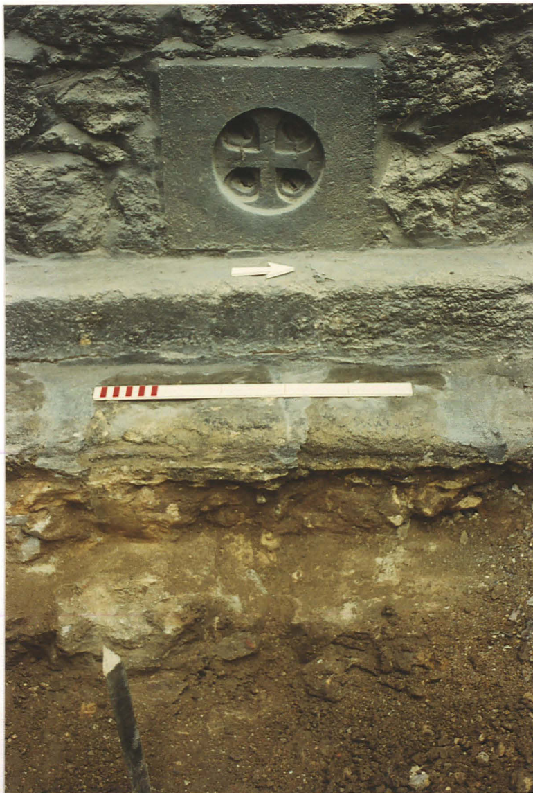
Pl. 6 Base of the east wall of the south transept, looking west, showing stepped out foundations; scale 50cm.
