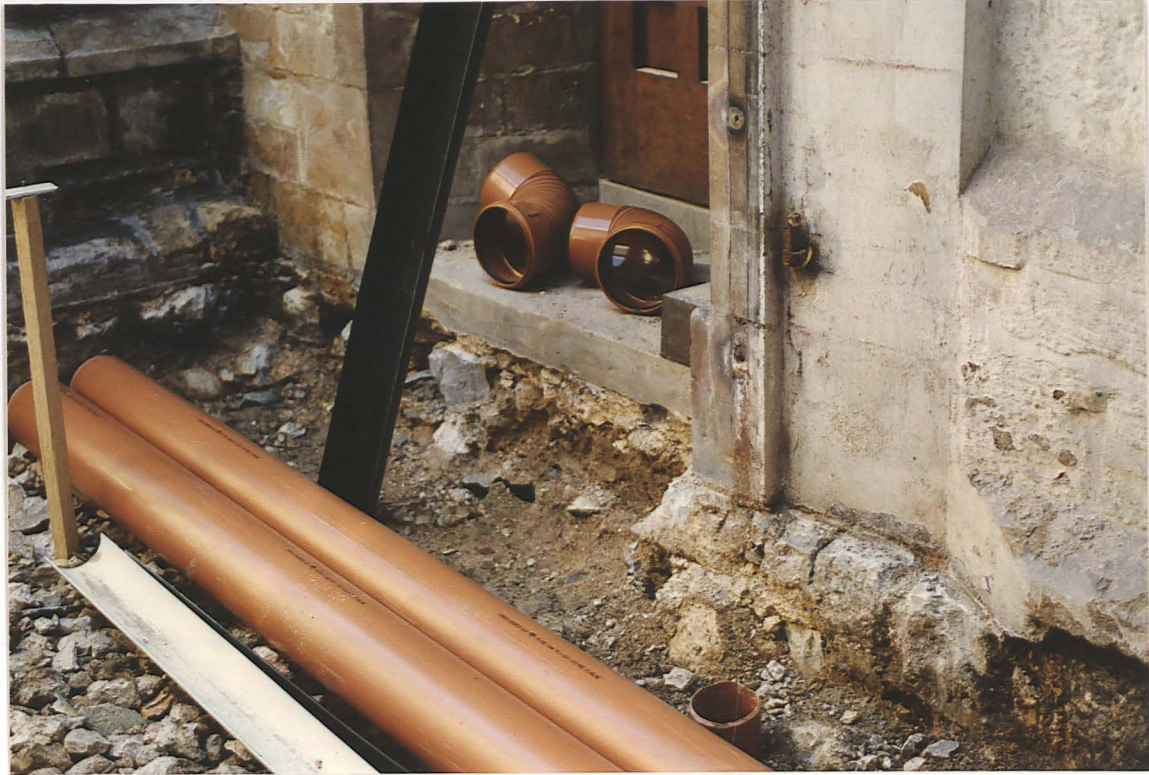
Pl. 3 North wall of St Thomas' Chapel, looking south-east, showing the door to the demolished passageway and the butress on the north-east corner of the building.
