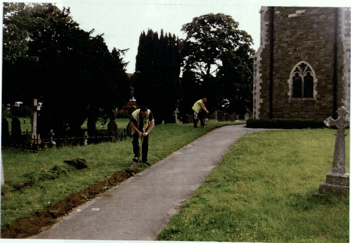
Pl. 2 Removal of turf (looking east).
