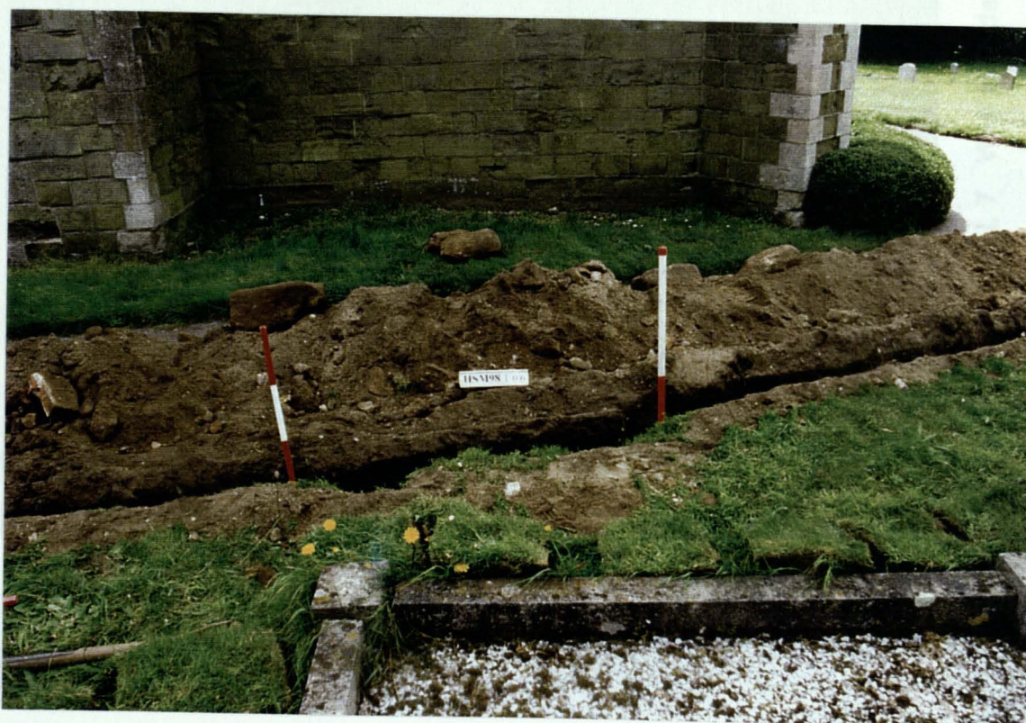
Pl. 6 Position of wall foundation 106, looking north (marked by red/white scales).
