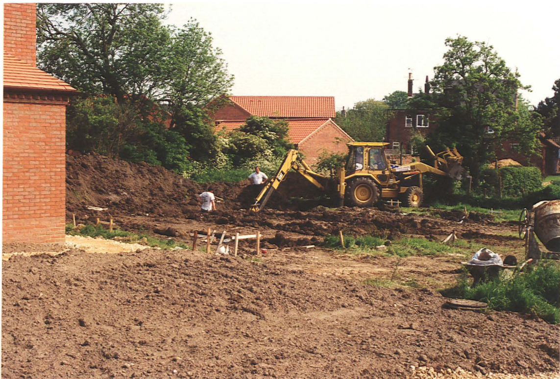
Pl. 2 Excavation of the foundation trenches (looking SE from beside Plot 1).
