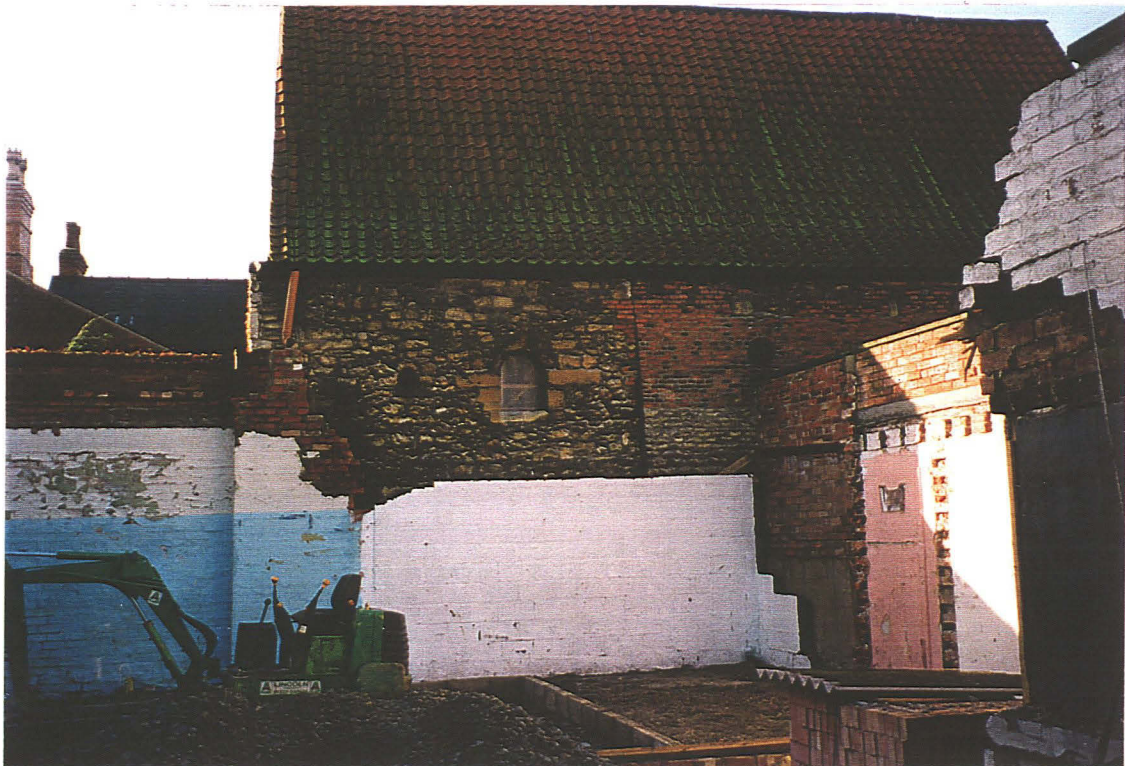
Pl. 3: View of the north face of the east range of the Guildhall as exposed following the demolition of the existing buildings (Compare with Pl. 1.).
