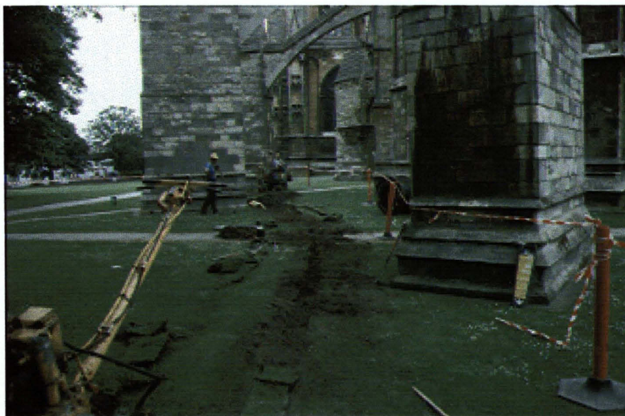
Plate 2 - View of the Cable Trench, adjacent to the Chapter House
