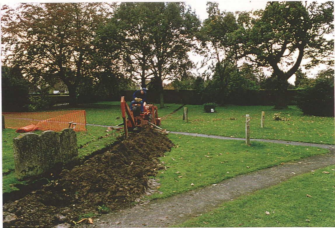
Pl. 1 View looking South of machine digging trench.
