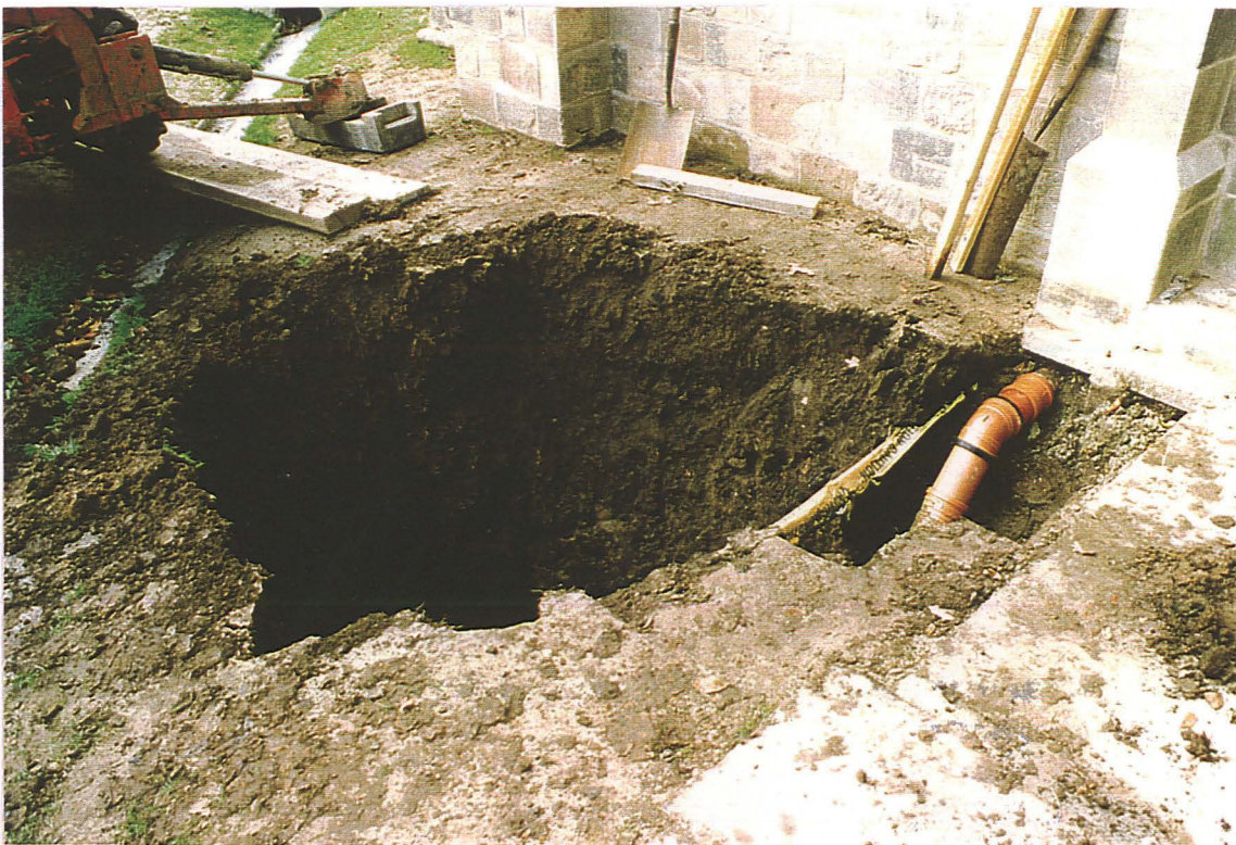
Pl. 4 Excavated area for junction box.
