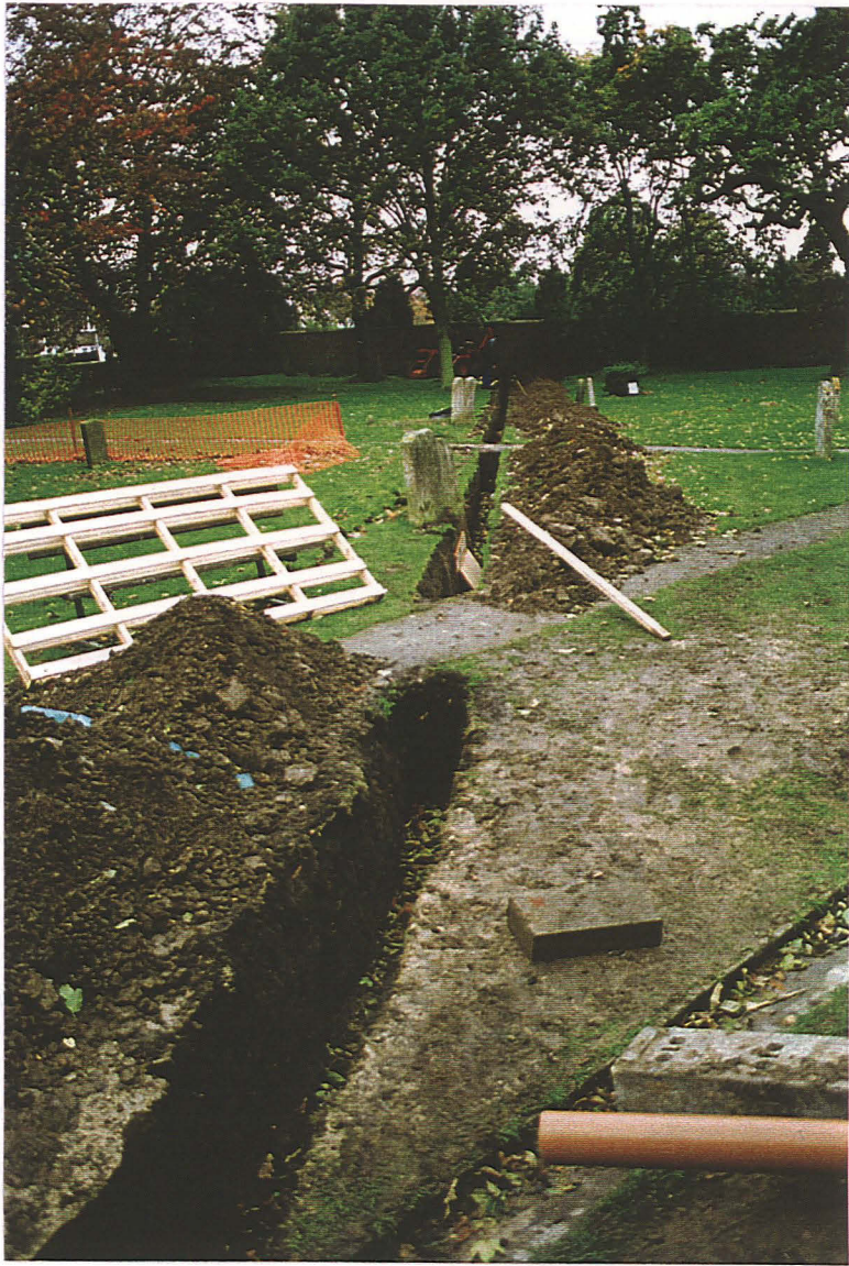
Pl. 3 Fully excavated trench looking South.
