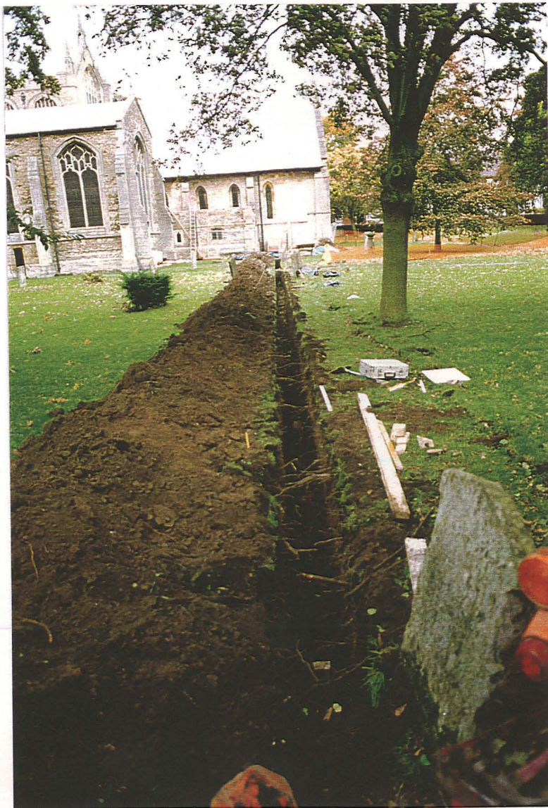
Pl. 2 Fully excavated trench looking North.
