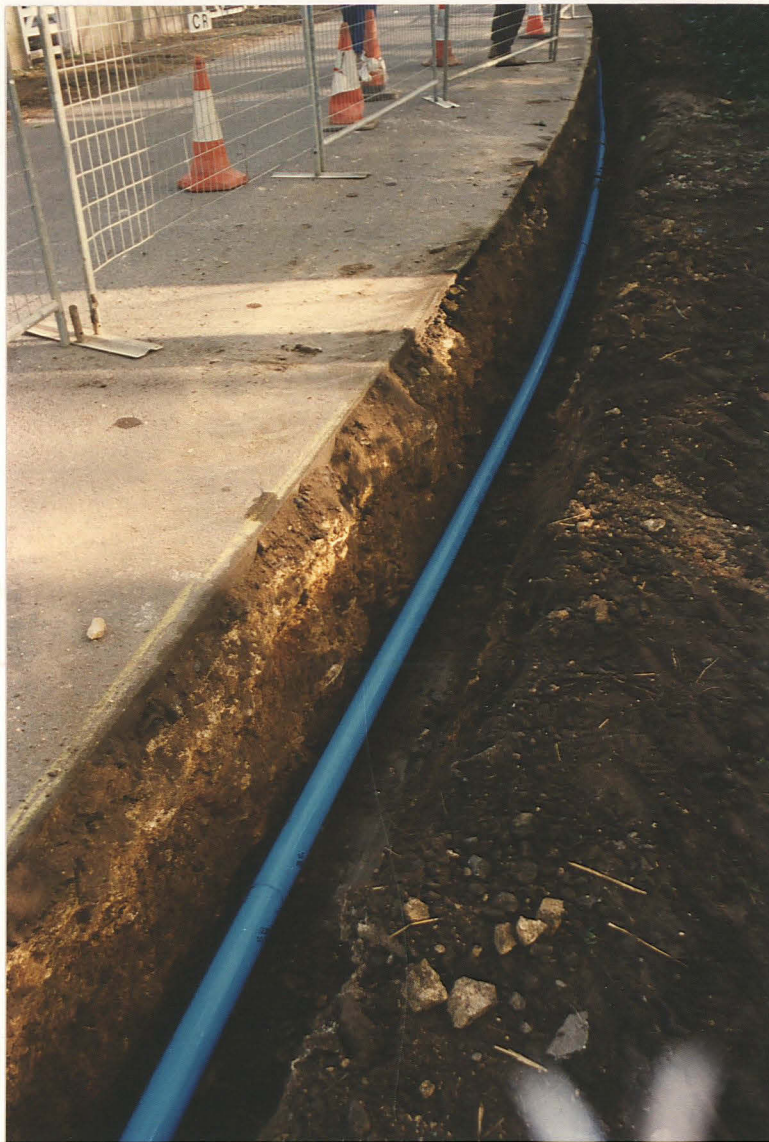
Pl. 18 Observation 21, looking east, showing continuation of organic silty deposits.
