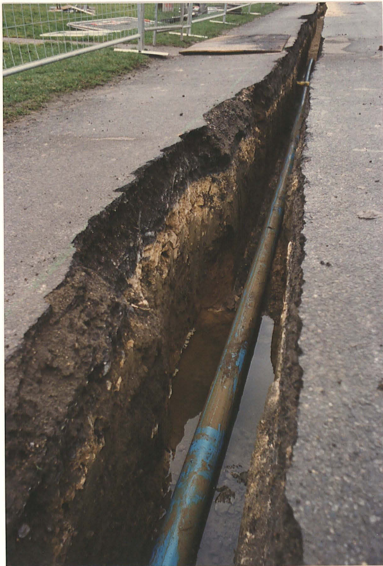
Pl. 1 Prince's Street, west of Princess Margaret Avenue. View looking west towards the Sleaford Road (B1188). Observation point 4 showing grey-brown clay/silt beneath road makeup of crushed limestone, probably part of a former watercourse.
