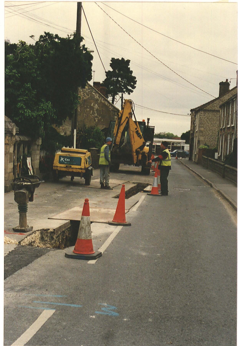
Pl. 1 Prince's Street, west of Princess Margaret Avenue. View looking west towards the Sleaford Road (B1188). Observation point 4 showing grey-brown clay/silt beneath road makeup of crushed limestone, probably part of a former watercourse.
