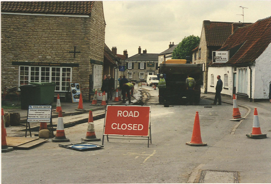
PI. 7 General view looking south along High St.
