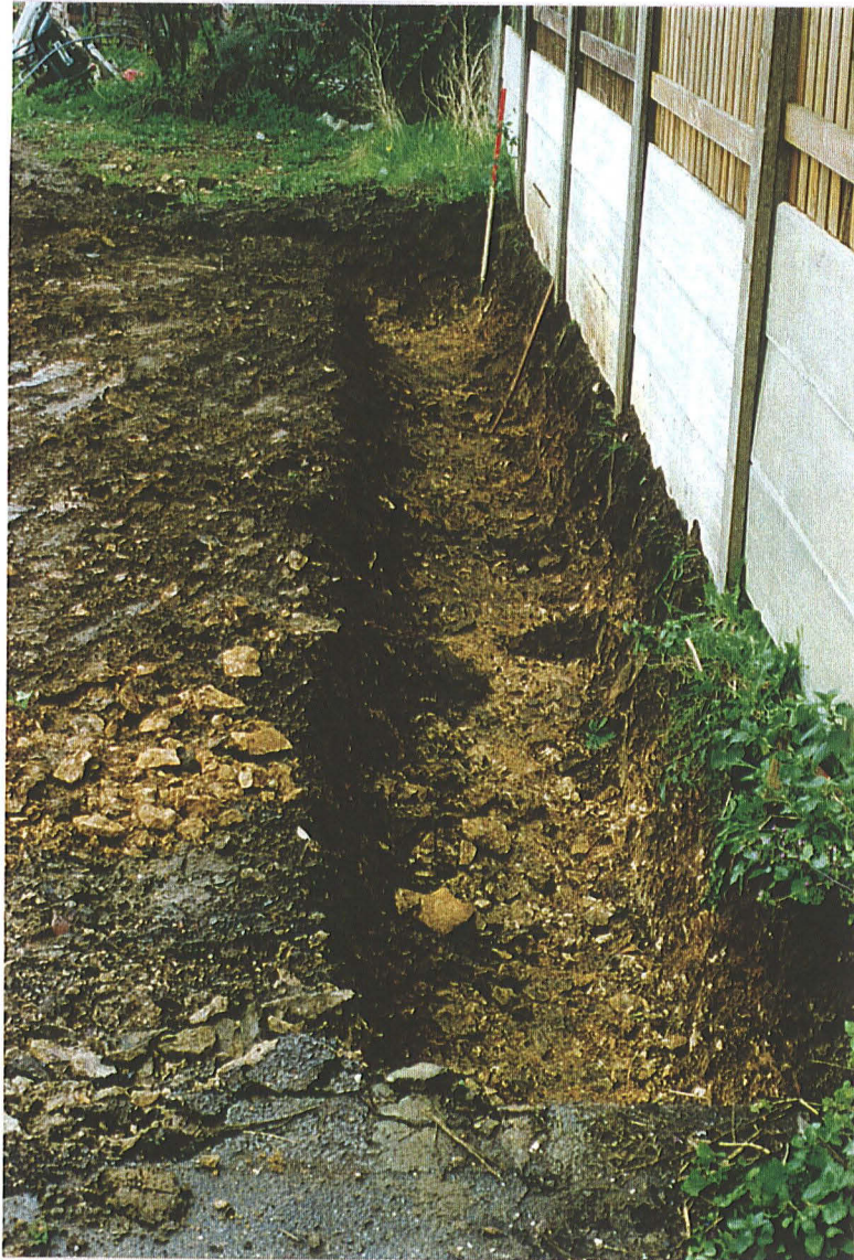
PI.3 Foundations for the garage western trench
