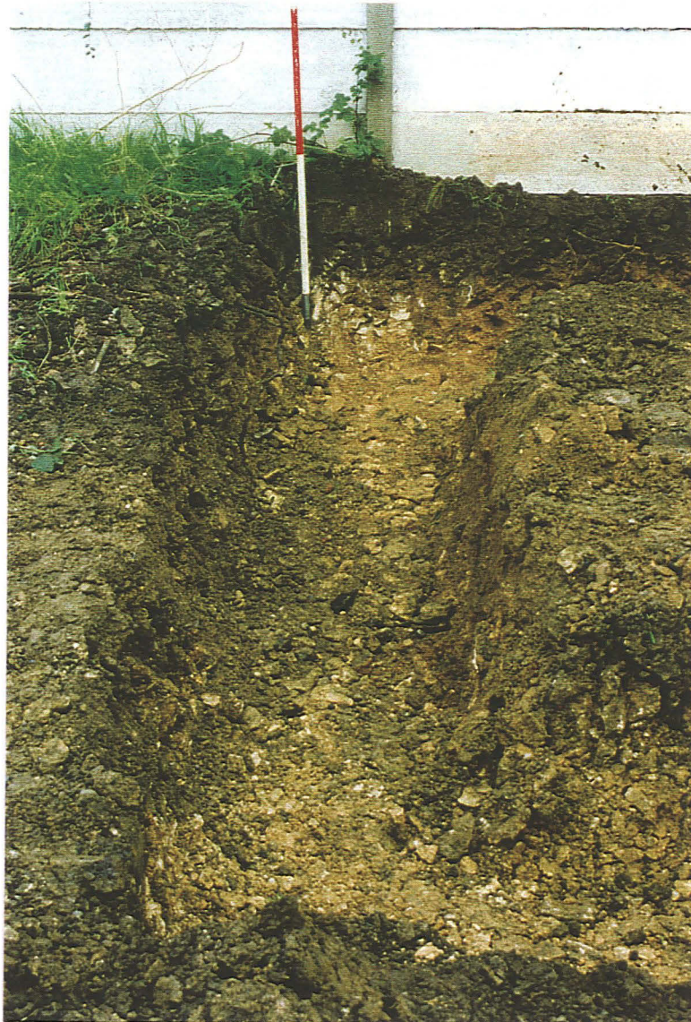
Pl.2 Foundations for the garage southern trench
