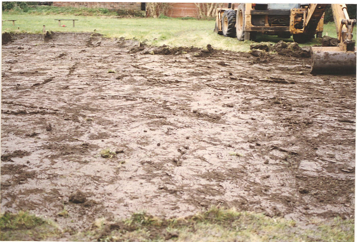
Pl. 2 Area of topsoil stripping looking north west.
