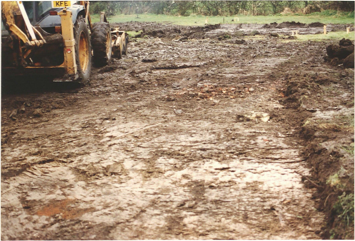
PI. 7 Area Stripped for access road
