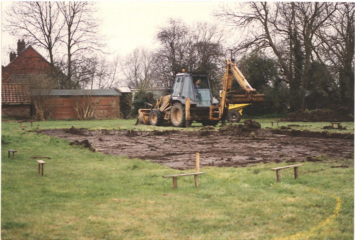
Pl. 1 General shot of development looking north-west.
