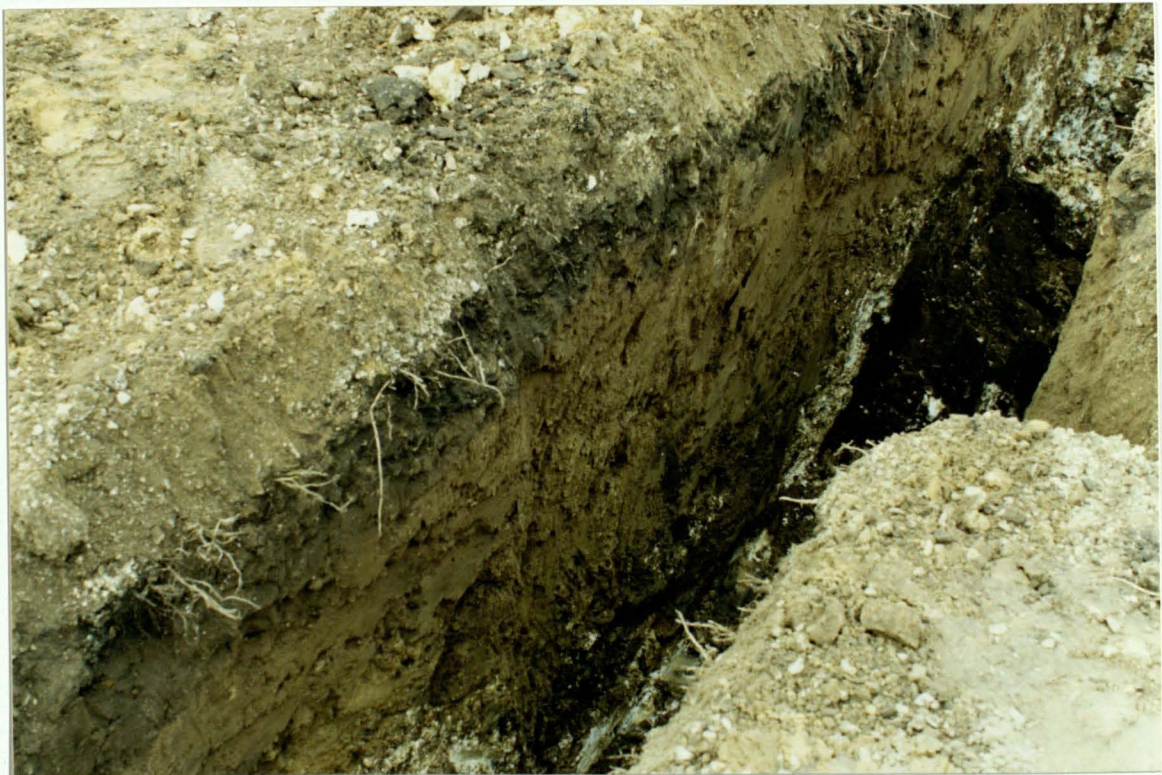
PI. 8 Pit 19 seen in west edge of foundation trenches for Plot 5 S , cut into chalk bedrock. Looking north.
