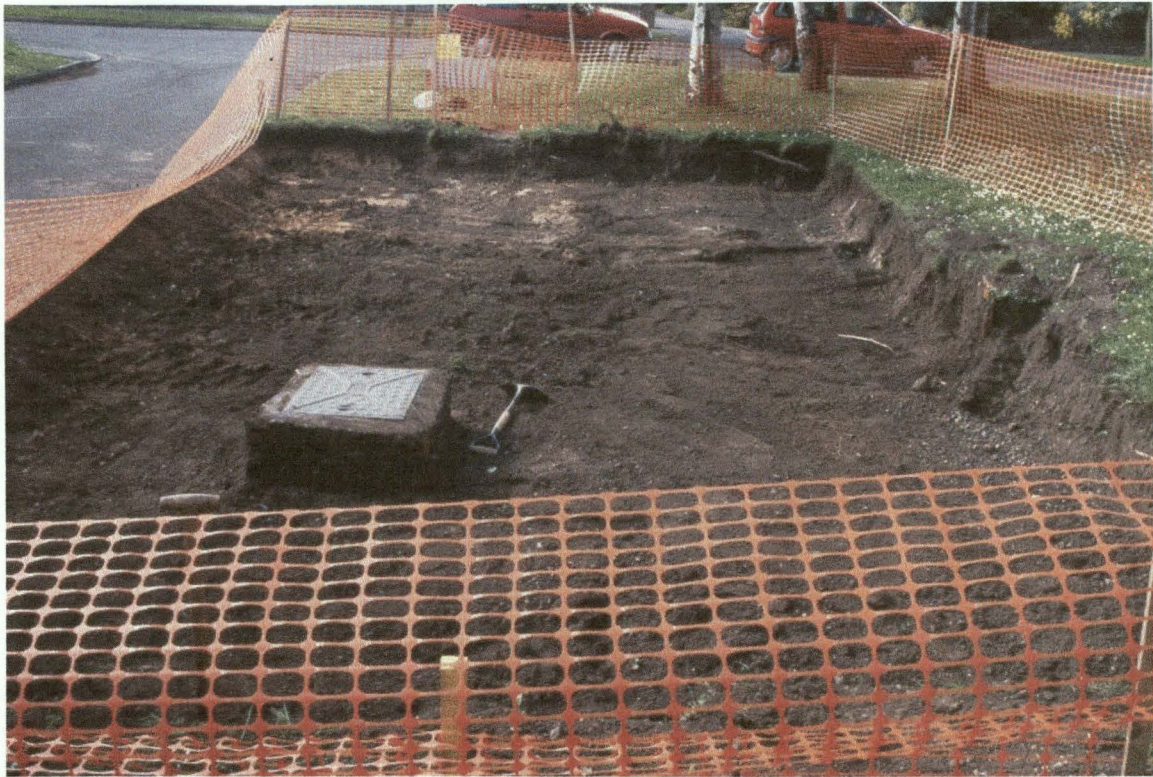
Plate 1: General view of the stripped compound area (looking south)
