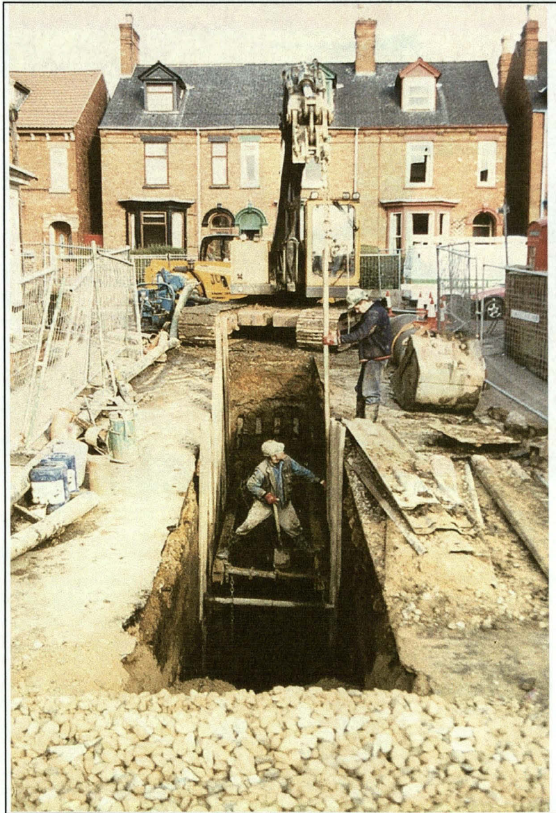
Plate 2: View of trenching in progress along Area 3 (Charles Street West)
