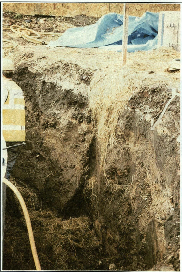
Plate 2: View of revealed deposits, Pumping Station site (Area 1)
