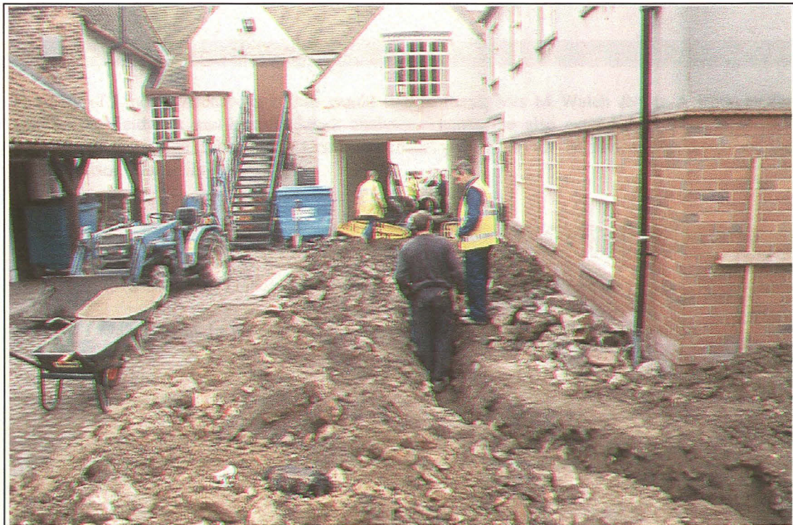
Plate II: General view of the combined service trench. Looking south towards Eastgate.
