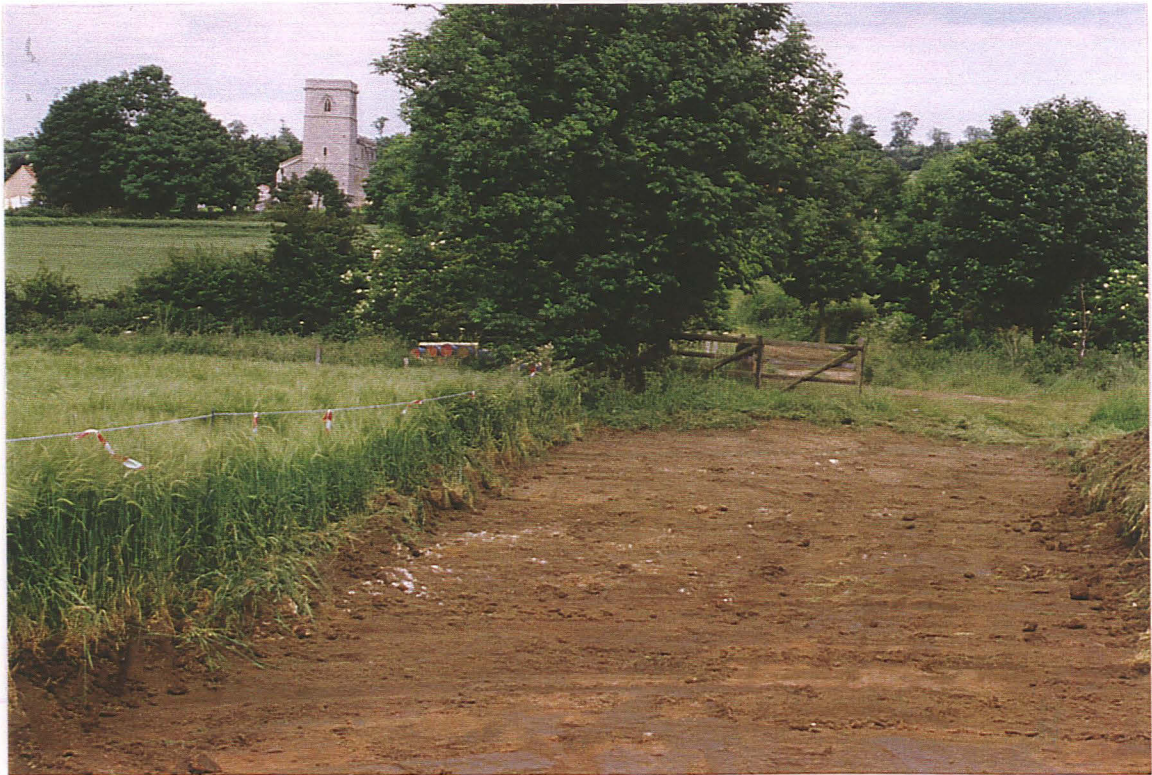
Pl. 11 Limestone and brick rubble at 2A, perhaps associated with demolished bridge beneath former railway line. Looking east.
