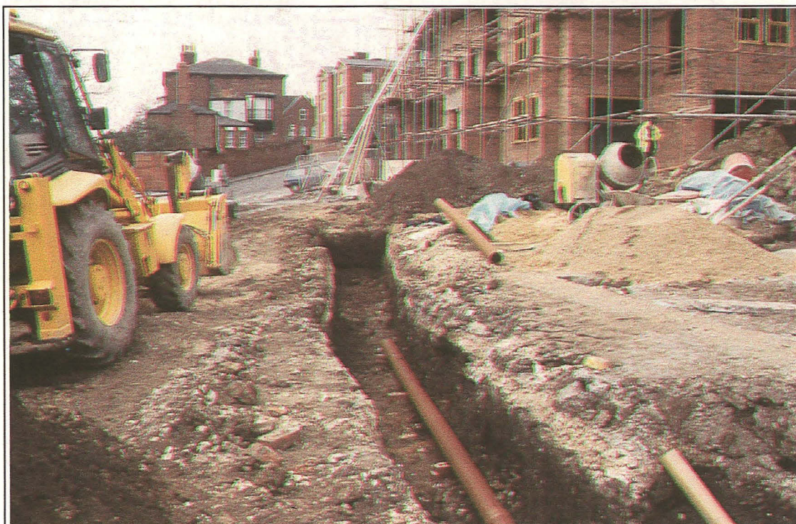
Plate II: The CST looking west towards Plot 1/2
