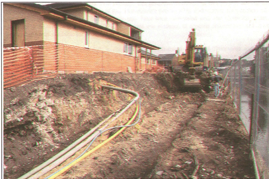
Plate I: General view of the medical centre as it nears completion. The exposed section in the foreground consists of recently deposited material laid down during the construction of the railway.
