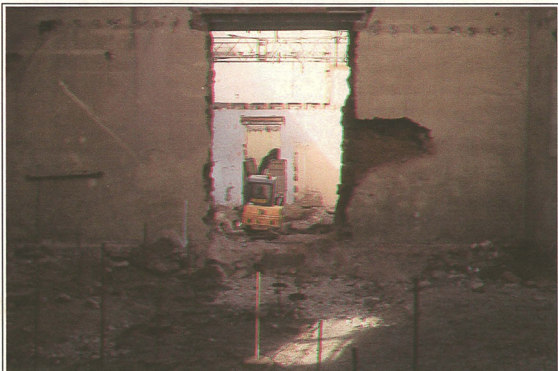
Plate II: View showing excavation of pile caps within building 2 (looking south).
