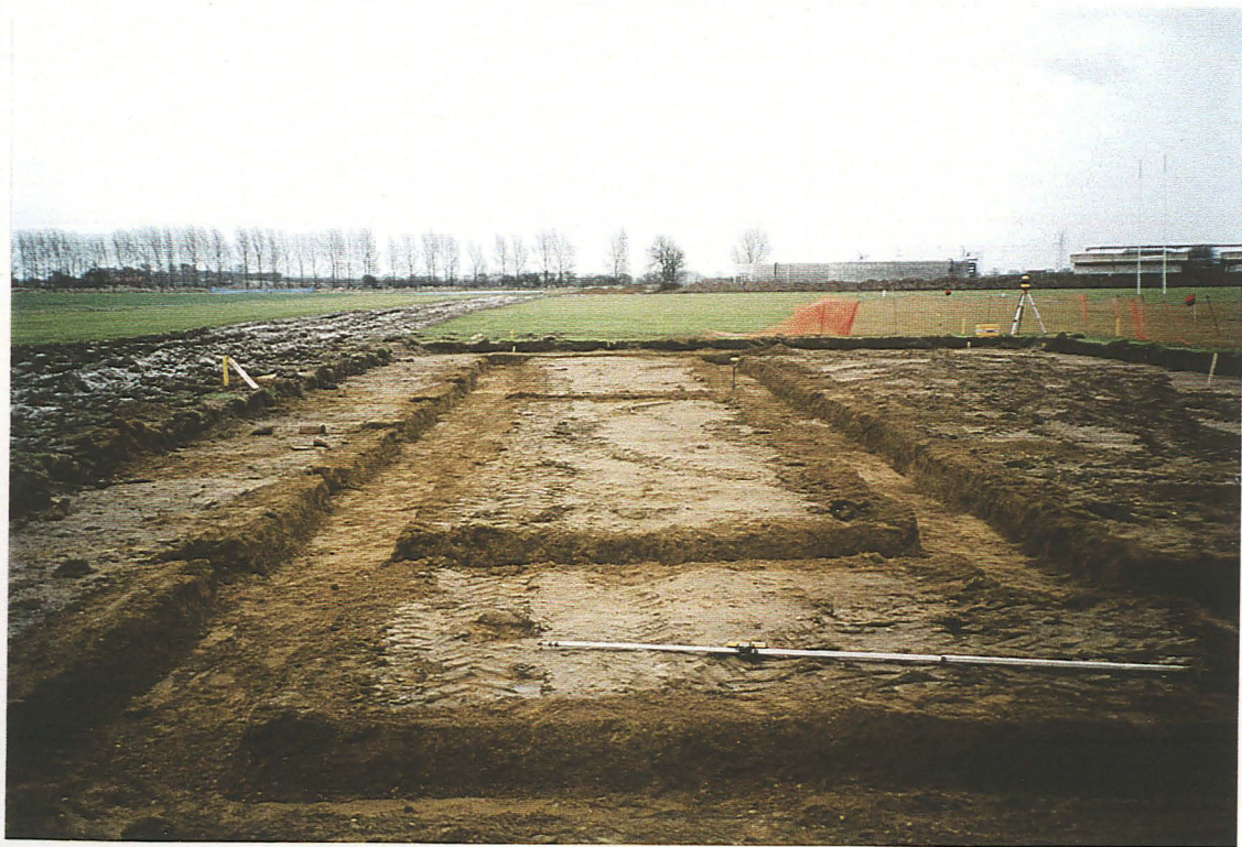
P.2 General view of incomplete pavilion footings, looking east.
