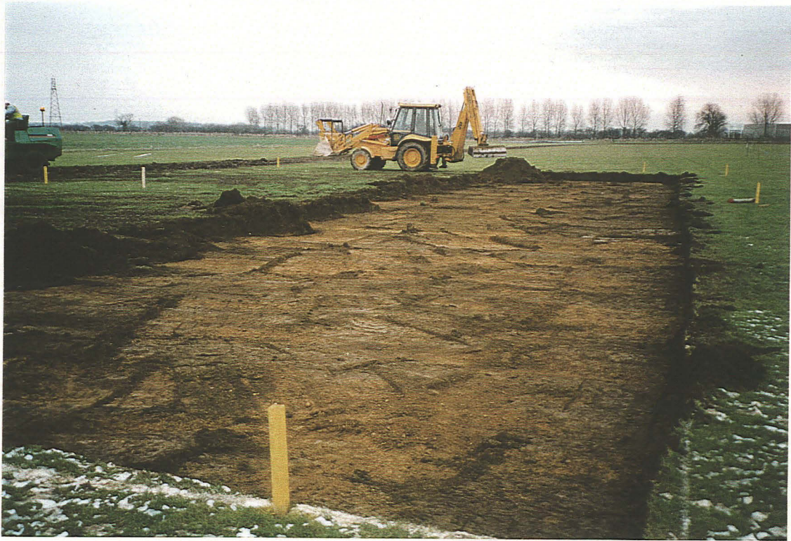
P.1 General view of topsoil strip for the pavilion, looking north-east.
