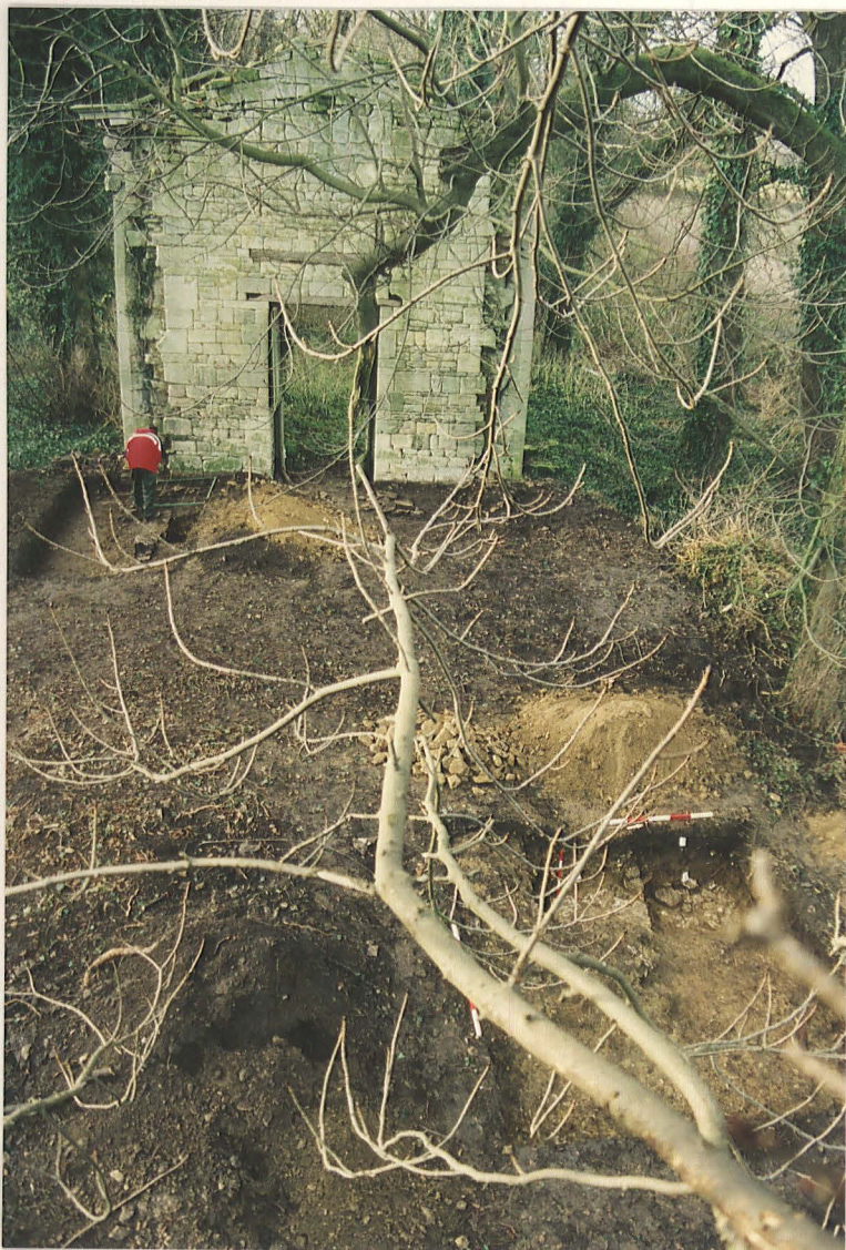
P1. Context view showing surviving facade, Trench 1 (background) and Trench 2 (foreground), looking west from above
