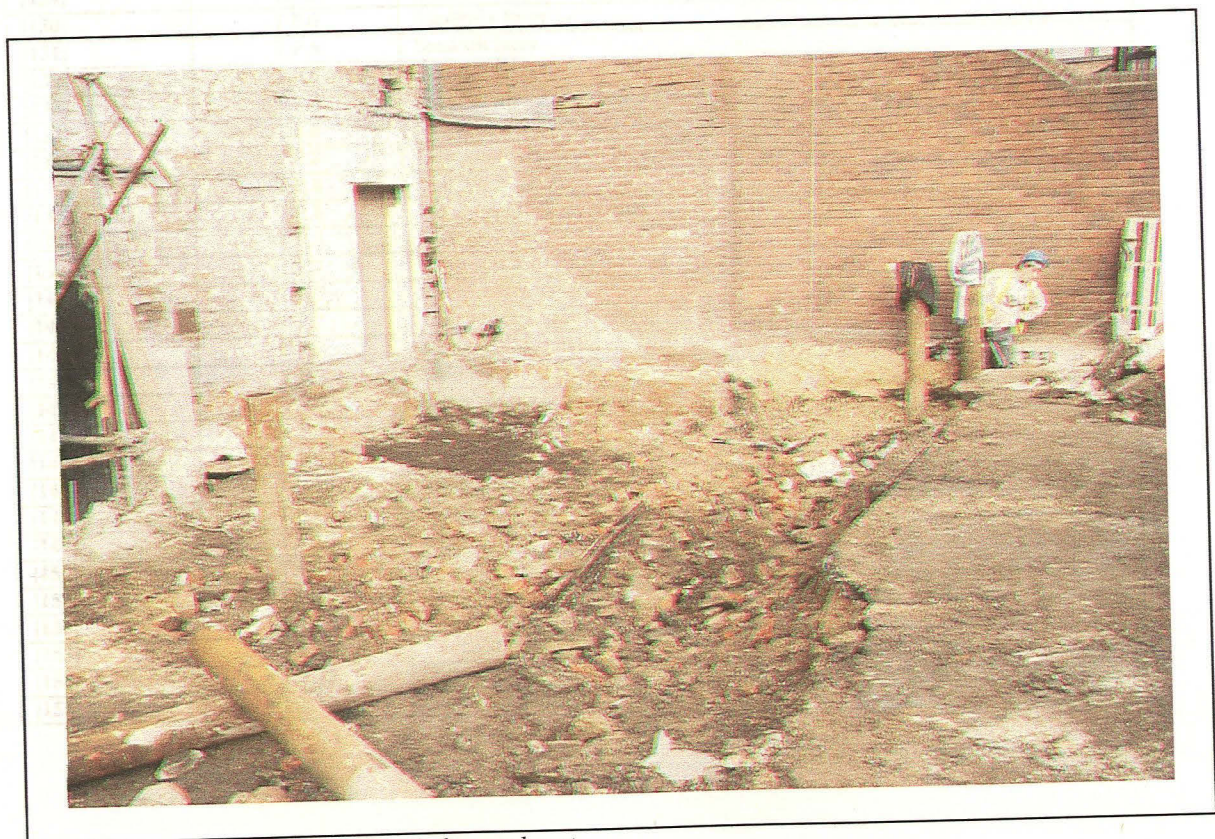
Plate 4: General view of rear yard area, looking north-west
