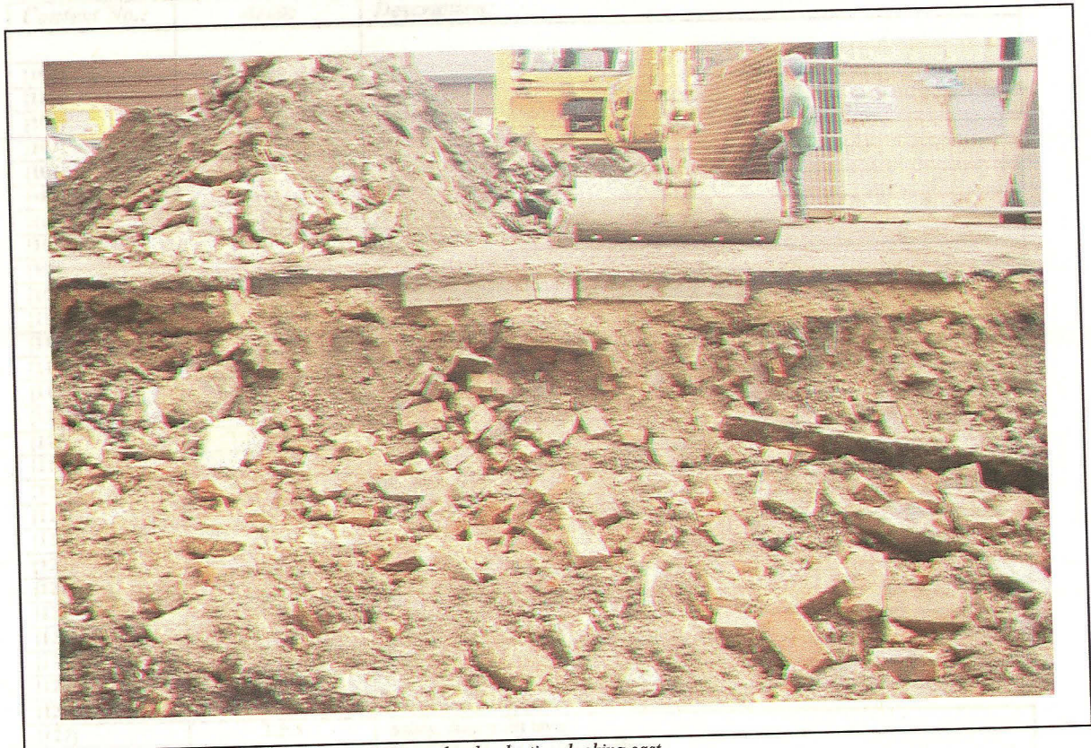
Plate 3: General view of rear yard area, following level reduction, looking east
