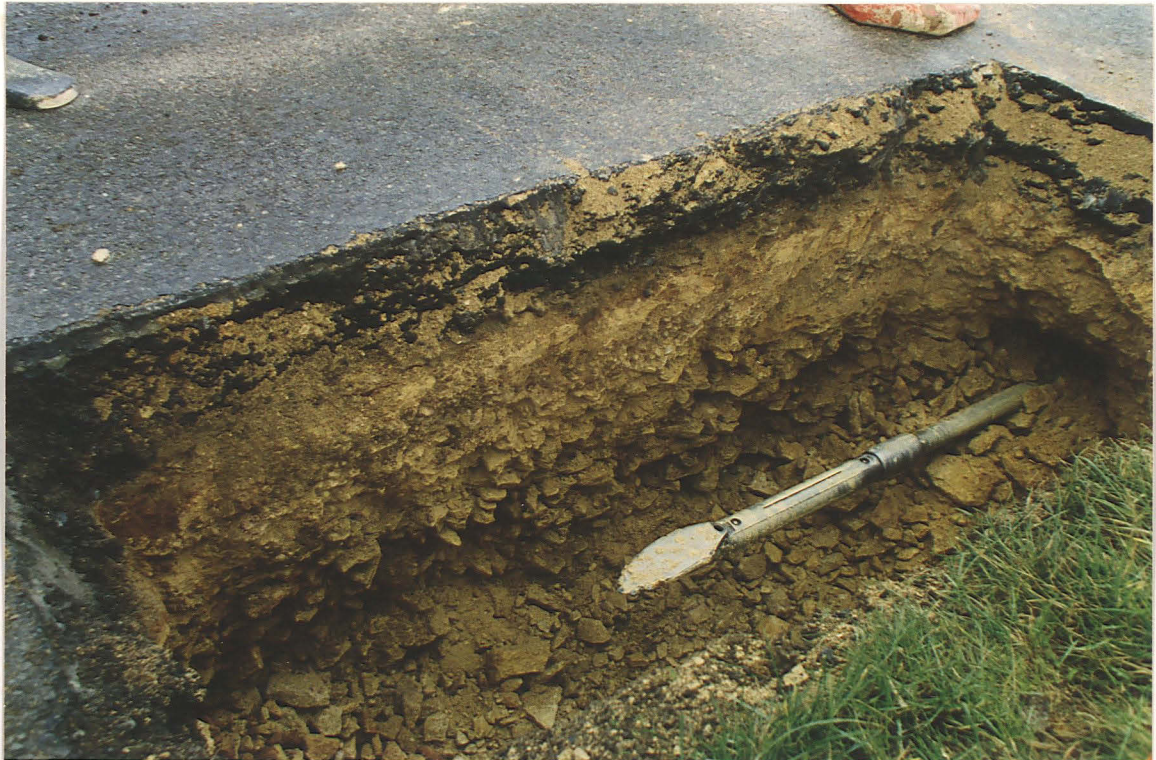
Pl. 8 Dense limestone bedrock in Trench 9.
