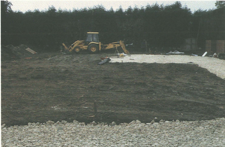
Plate 1: General view of the site, looking north
