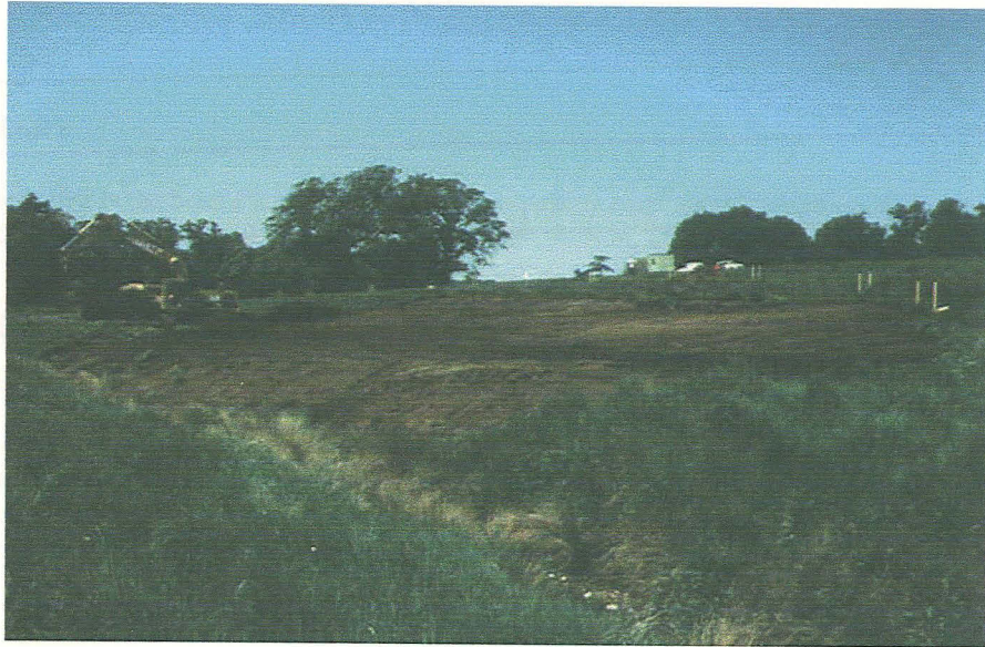
Plate 1: General view of the topsoil stripping, looking northwest
