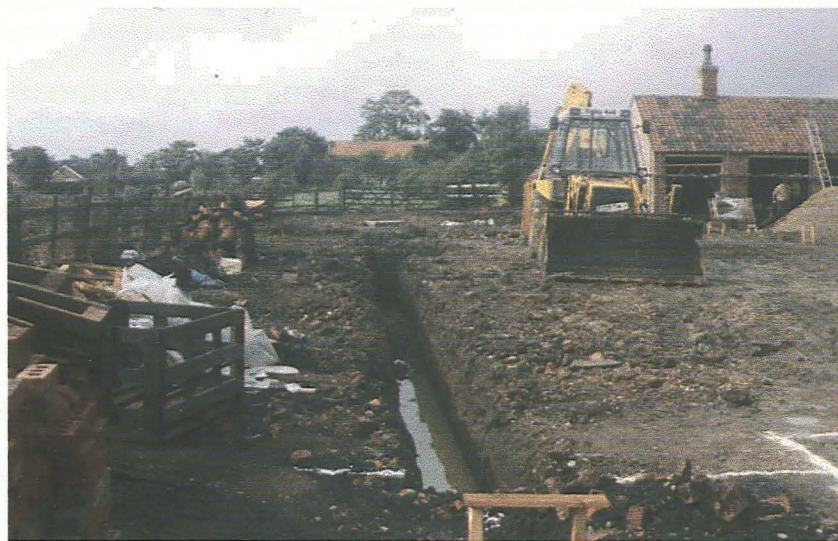
Plate 2 - General view of the site, looking north, showing the foundation trenches
