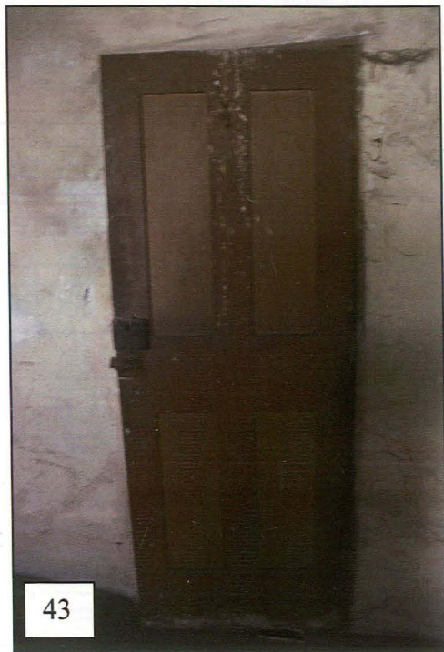
The door to Room 6 appeared to be of original 18 th century date: it was of plain four-panel type, 1½" in thickness, with a thumb-latch and lever lock.
