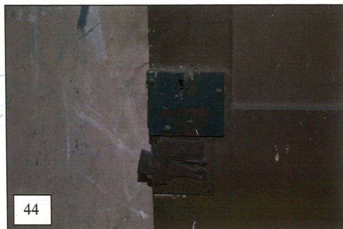
The door to Room 6 appeared to be of original 18 th century date: it was of plain four-panel type, 1½" in thickness, with a thumb-latch and lever lock.
