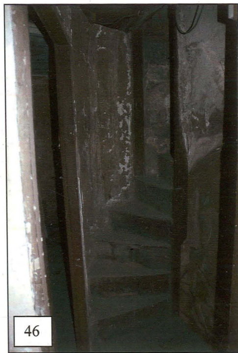
A 180° winding staircase gave access to an attic room. The staircase was of ¾" timber with a rise of 7¾" and treads of between 10 and 11" (narrowing to 2" at the newel). The staircase was divided from Room 7 by a curved wall of 10"-11" x 4¼" stretchers laid on edge to produce a 3" thick wall. The walls and partitions were all plastered; the soffit of the stairs was of plaster and lath. In the area of the second floor landing, the floor was of 8" plain boards, ½" in thickness and laid east-west.
