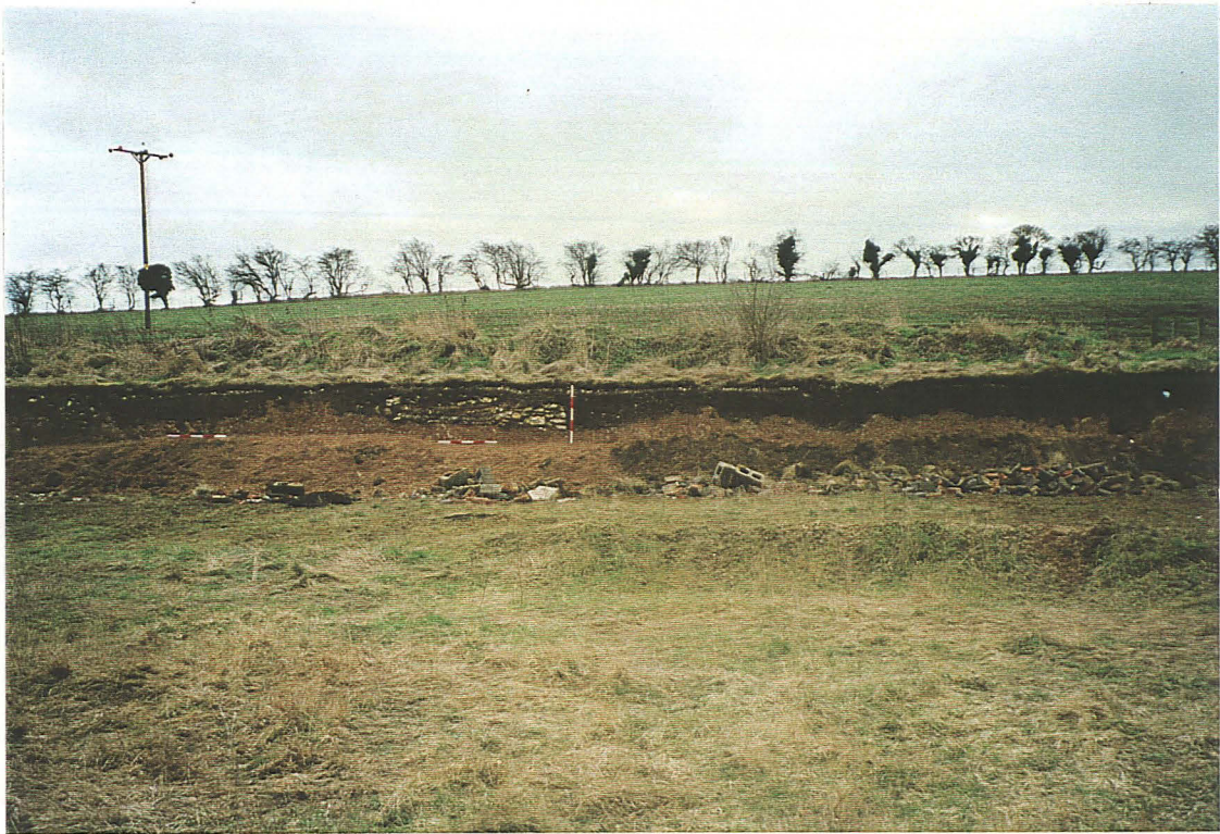
P.1 General view of the site showing the lime kiln, looking south.
