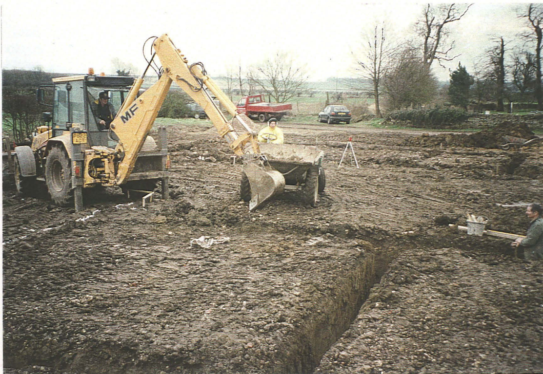
P.1 General view of the foundation trenching in progress, looking south.
