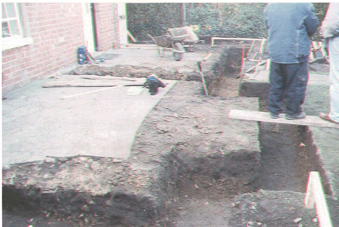
Plate 1: General view of site, following foundation trenching - looking west
