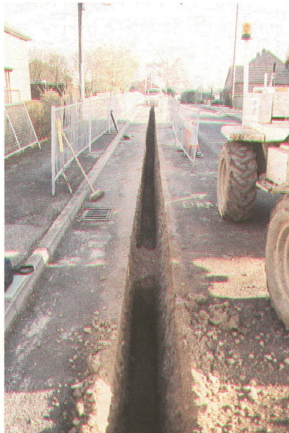
Plate 2: General view of Area B trench - looking east
