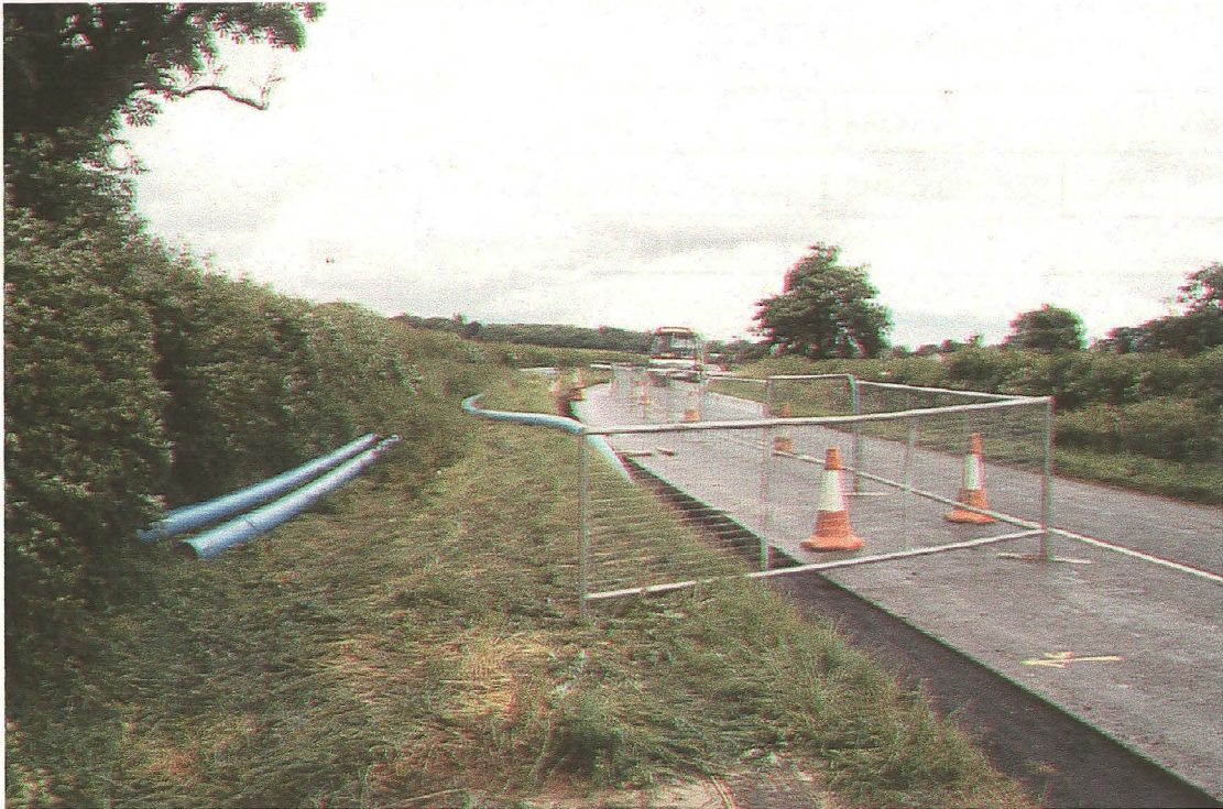
Plate 1: General view of Area A trench - looking east
