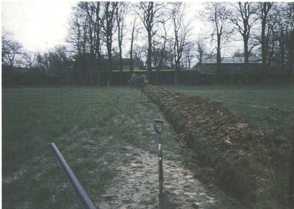
Plate 1 - The cable trench, looking west towards Brackenborough Hall
