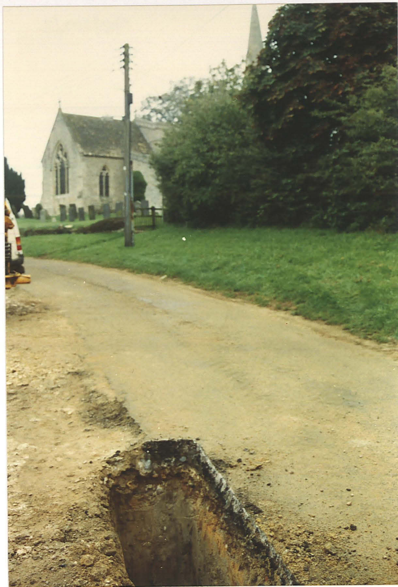
Pl. 1 Position of Trench 1 (looking SW to St. Mary Magdalen's Church).
