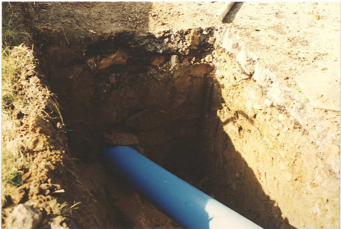
Pl. 9 Post-medieval road foundation above clay, Trench 3, Lenton-Pickworth Road.
