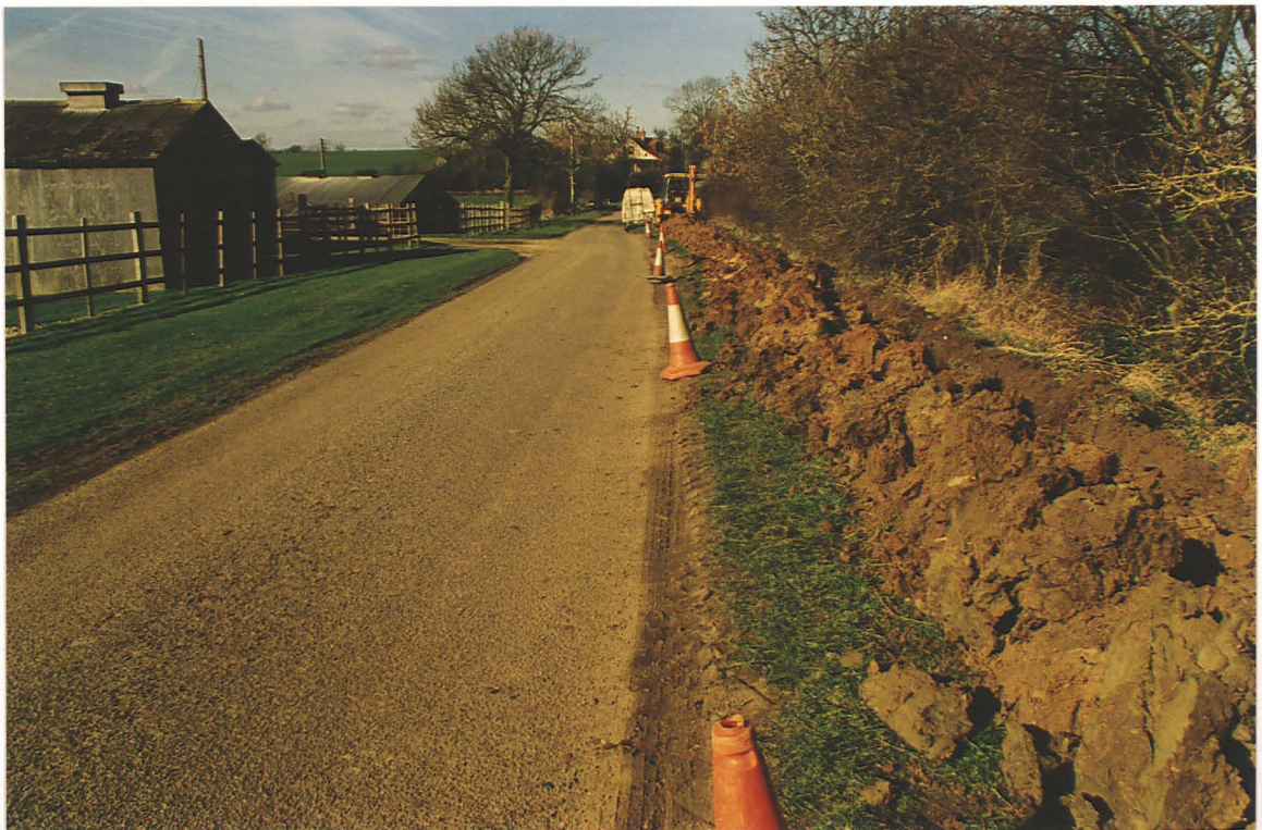
Pl. 2 Position of the trench near the poultry farm, Hanby (looking north).
