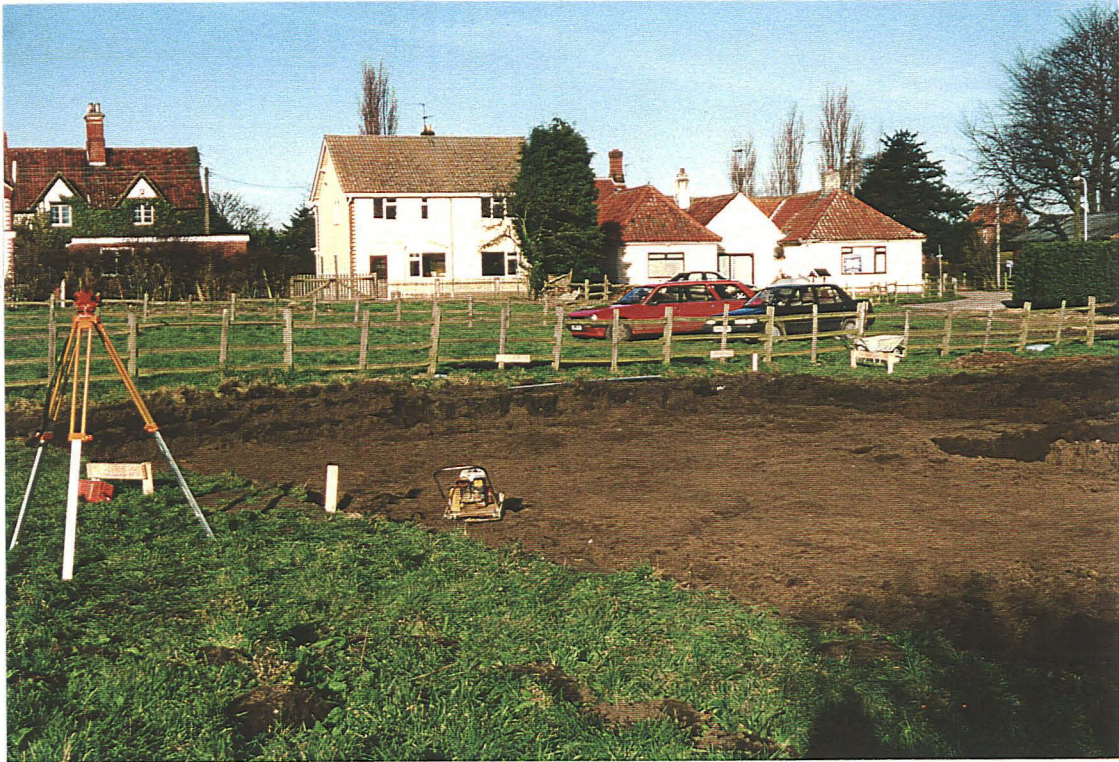
P1. General view of house footprint following excavations, looking north-west
