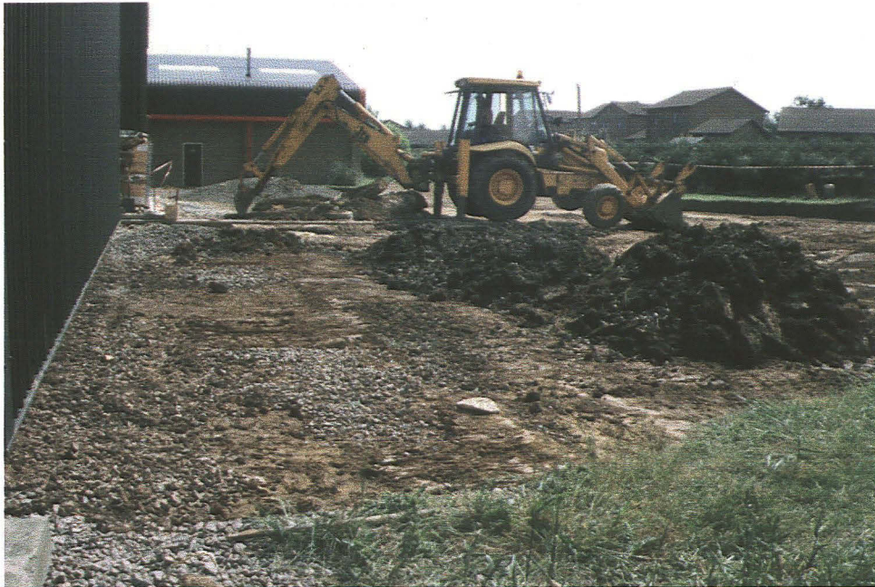
Plate 1 General view of site, looking north
